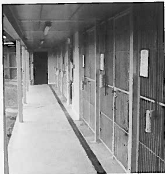
Protected external runs (showing drainage)
